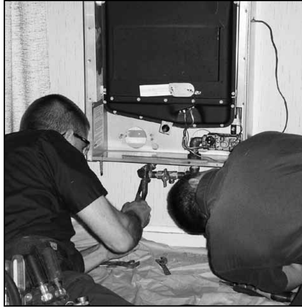
Our installation team - Chris and Norm
